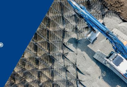
When faced with soft foundation soils where expensive piling and other deep ground improvement solutions are not viable or too costly, the TensarTech® Stratum® Cellular Foundation Mattress System provides an alternative approach for construction, often delivering savings in cost and time.
