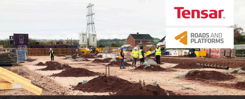
Areas of weak ground meant some homes were piled, requiring a large temporary working platform to provide a safe working area for the piling rig.
